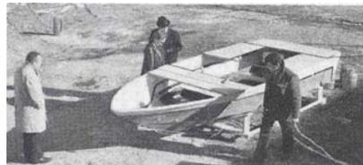
Fully instrumented boat hull. Over 50 thermocouple wires are connected to multi-channel recorders.
